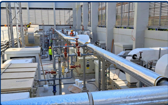
Pre-Insulated Ductwork — Rooftop Commercial Sector, KSA
